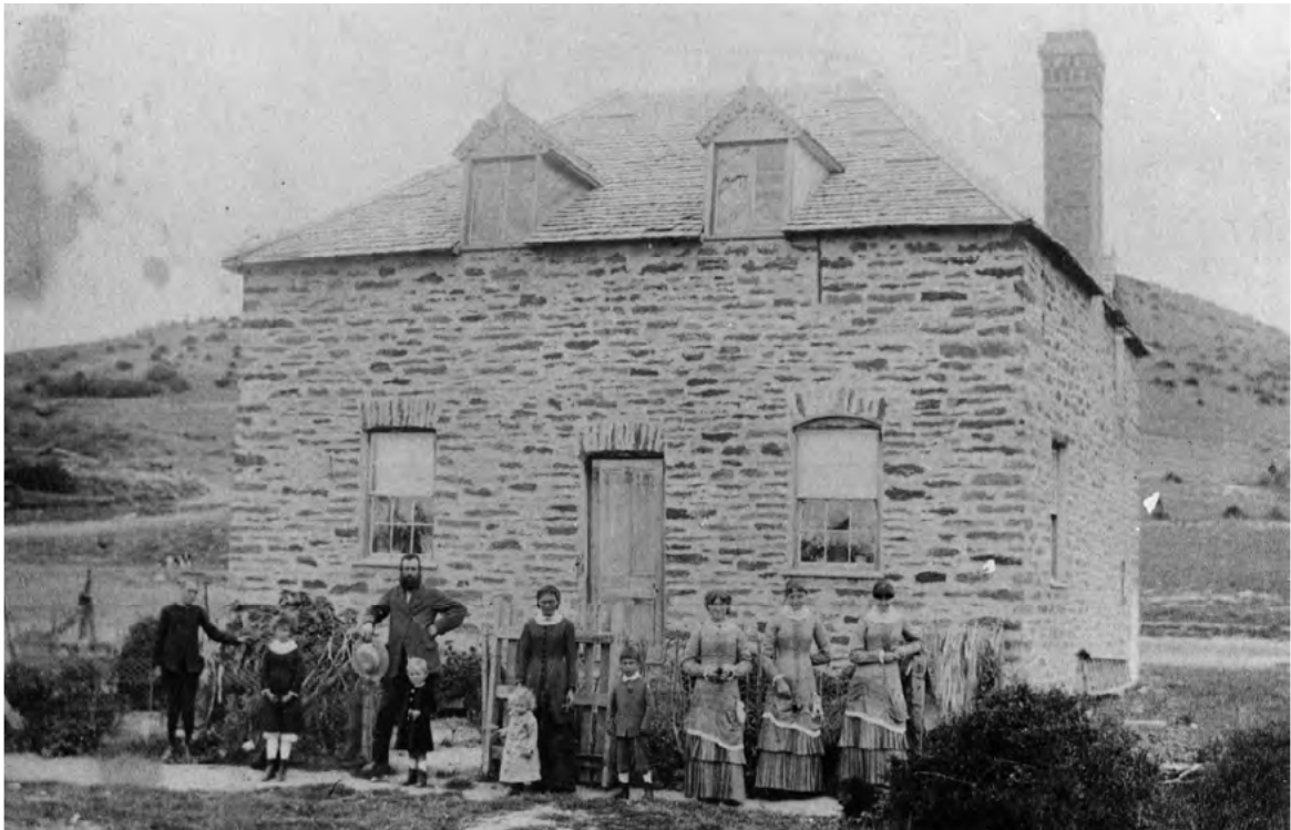
1. John Butler and family, 1885 (Hocken Library, Photograph Collection 80/217) . Note the shingled roof, now replaced by corrugated iron. In addition, the chimney is no longer fully intact and the small enclosing wall at the northeast corner was added later. The building appears to be largely unchanged since this photograph was taken.
