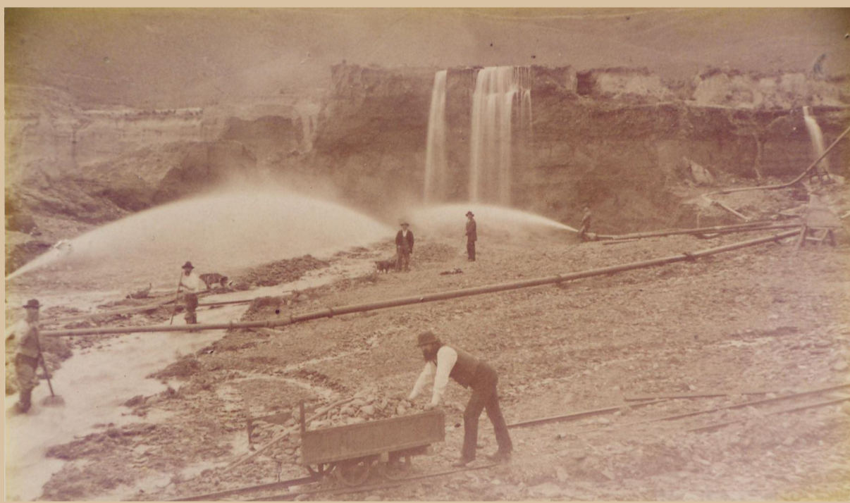
Gold sluicing at Drybread © MAF
